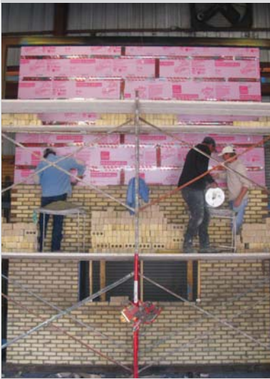
NFPA 285 test wall under construction.
