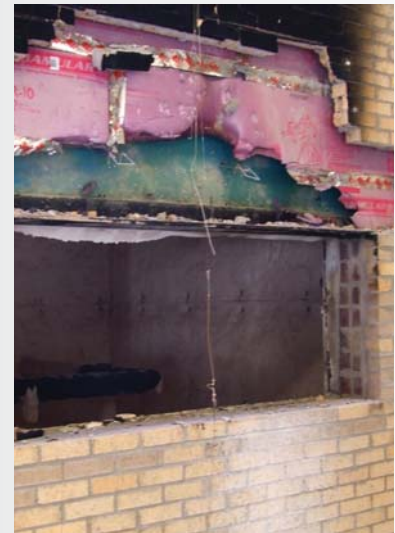
FOAMULAR® XPS with brick veneer stripped away above the test window showing limited damage and minimal fire spread after the NFPA 285 fire test.
